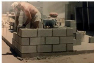
David starting to build the addition on our house in AZ. (1986)
