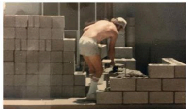
David building the addition on our house in AZ.
